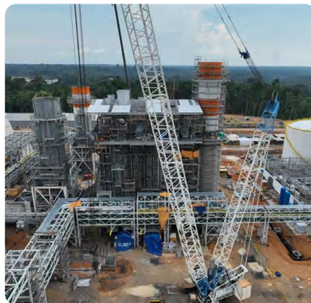
Assembly of pipe rack modules for Azulão 950; in total, there are 18 carbon steel components weighing 354 tonnes, equivalent to the weight of nearly 250 compact cars
